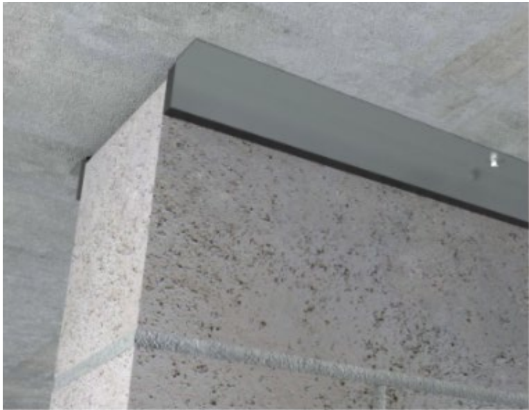
Masonry isolator bracket
