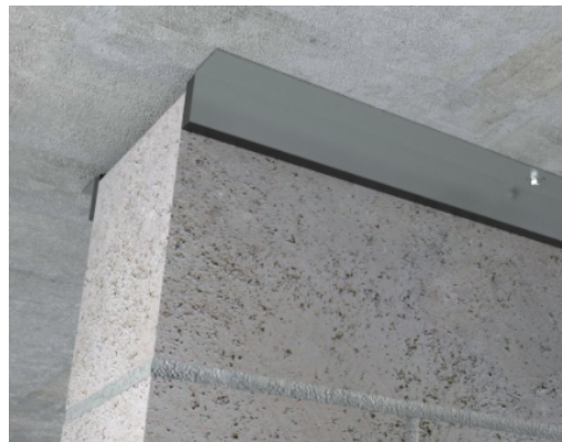
Diagram 2.3.12 : Masonry isolator bracket
