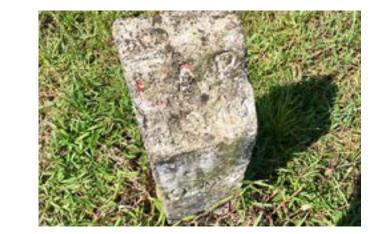
STONE MARKER INDICATES A 400MM DIAMETER GALVANIZED WATER PIPE BY THE LEMBAGA AIR PERAK (LAP) BELOW THE GROUND LEVEL. (lembaga air perak,
